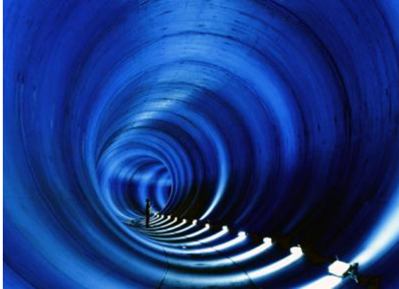
Figure 64 - The huge DTSS pipes from inside.
