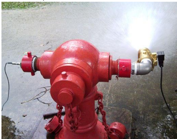
Figure 38 - Emulation of a burst water main was quickly detected by a neighbouring sensor node of Singapore's prototype monitoring network.
