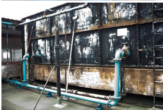
Figure 42 - (Up) Tapping for down-comers in PP-R (Down) New lines laid alongside old lines to facilitate uninterrupted supply during replacement.
