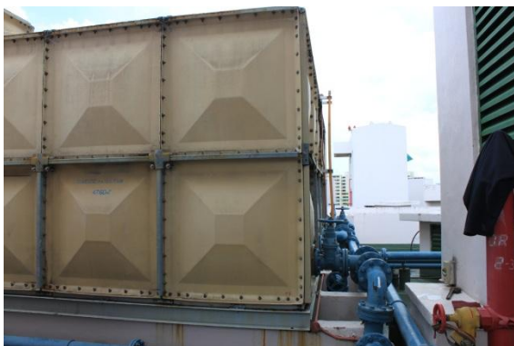
Figure 41 - The Domestic Water Storage being cleaned.
