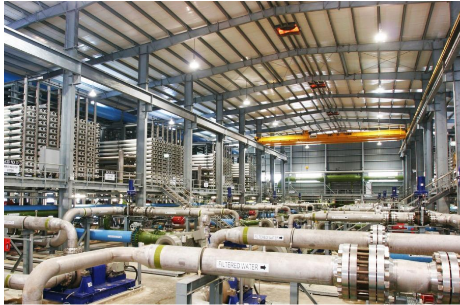
Figure 74 - The Seawater Reverse Osmosis Building at Tuas (Source; Hyflux)
