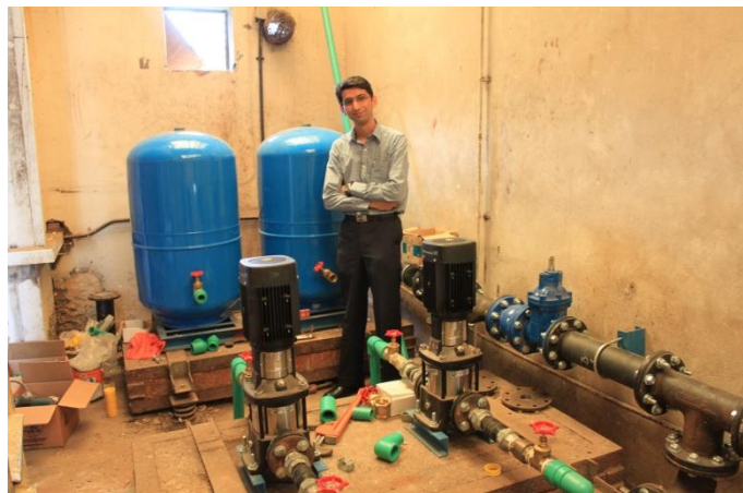
Figure 40 - In the Pump Room during a retrofit installation.
