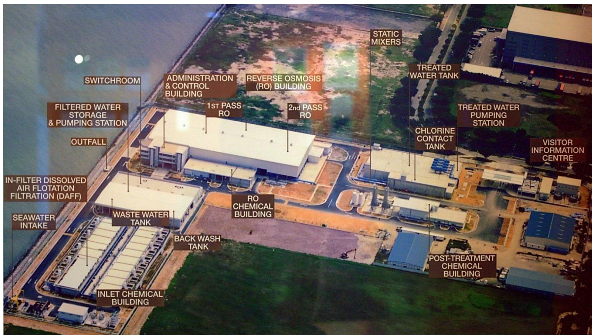
Figure 73 - An Aerial view of SingSpring Plant at Tuas. (Source – Hyflux)
