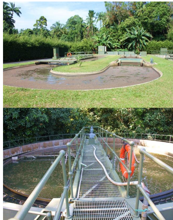
Figure 36 - The Sewage Treatment Plant of the Zoo.
