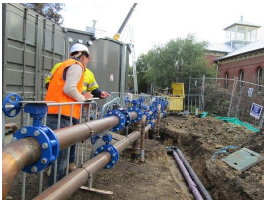
Pure water tank of Bendigo Hospital process of plumbing
