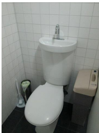
Bathroom toilet with wet sink attached
