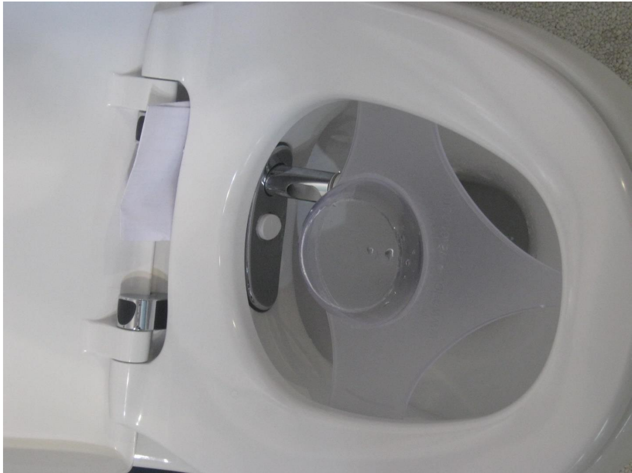
Figure 24: WC with apparatus as bidet
