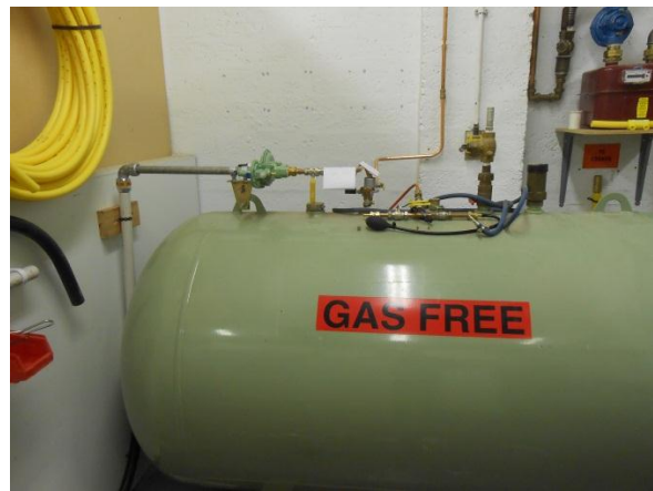
Simulated LPG tank installation
