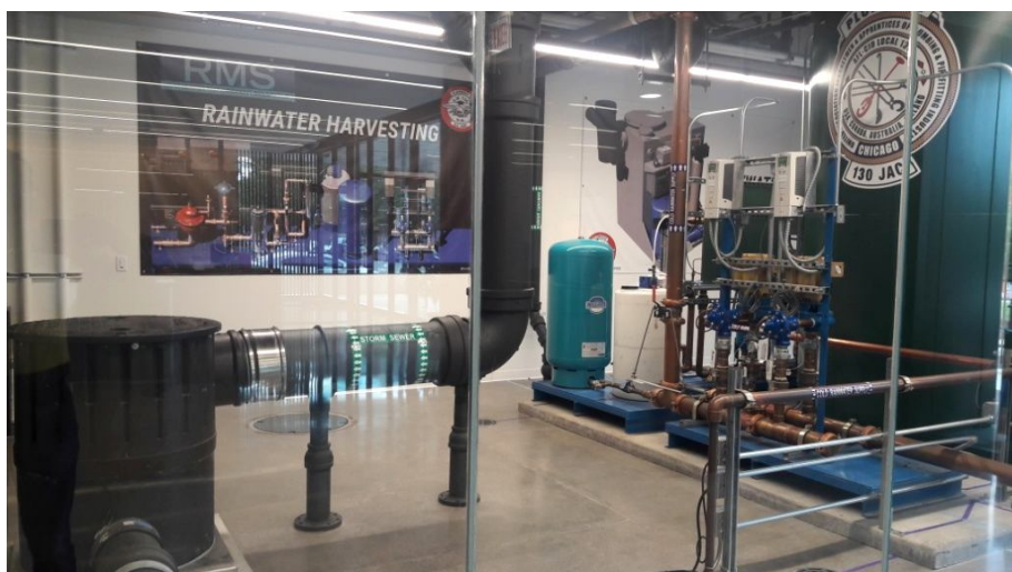
Rain water harvesting system at Local 130
