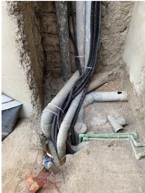
Figure 13 Soil, waste and water lines. The line with a hole on top of the pipe was connected to a future water closet.
