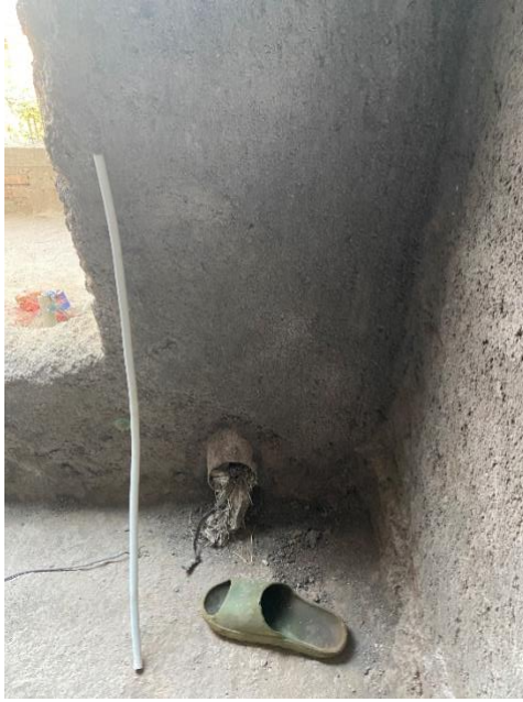
Figure 14 Water closet connection to back outlet water closet.
