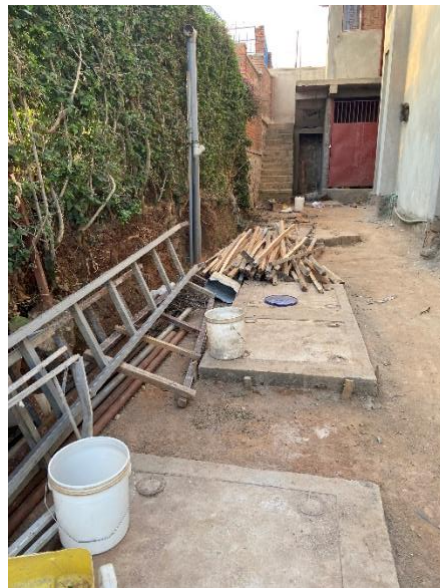
Figure 15 Sewage collection tanks. Tanks are pumped on a periodic schedule. A vast majority of Rwanda residential, commercial and industrial structures do not have access to public sewer systems and sewage treatment facilities.
