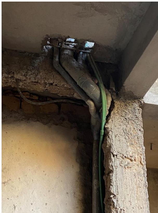
Figure 11 Soil stacks, waste stacks and water risers.
