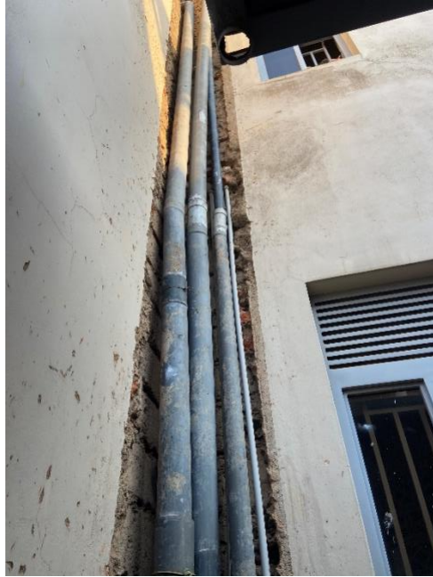
Figure 12 Soil and waste stacks.
