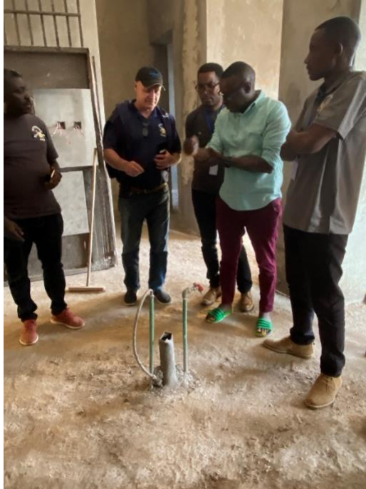
Figure 10 Bigley explains to the owner and members of the RPO the differences in accepted plumbing practices in North America compared to what he was seeing on site. This was the kitchen Sink rough in.
