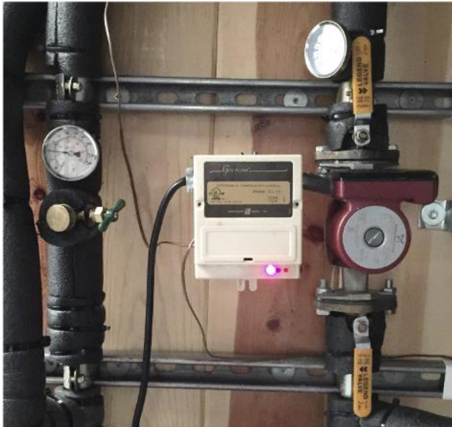
(Pumps and thermometers to control the system) 24
