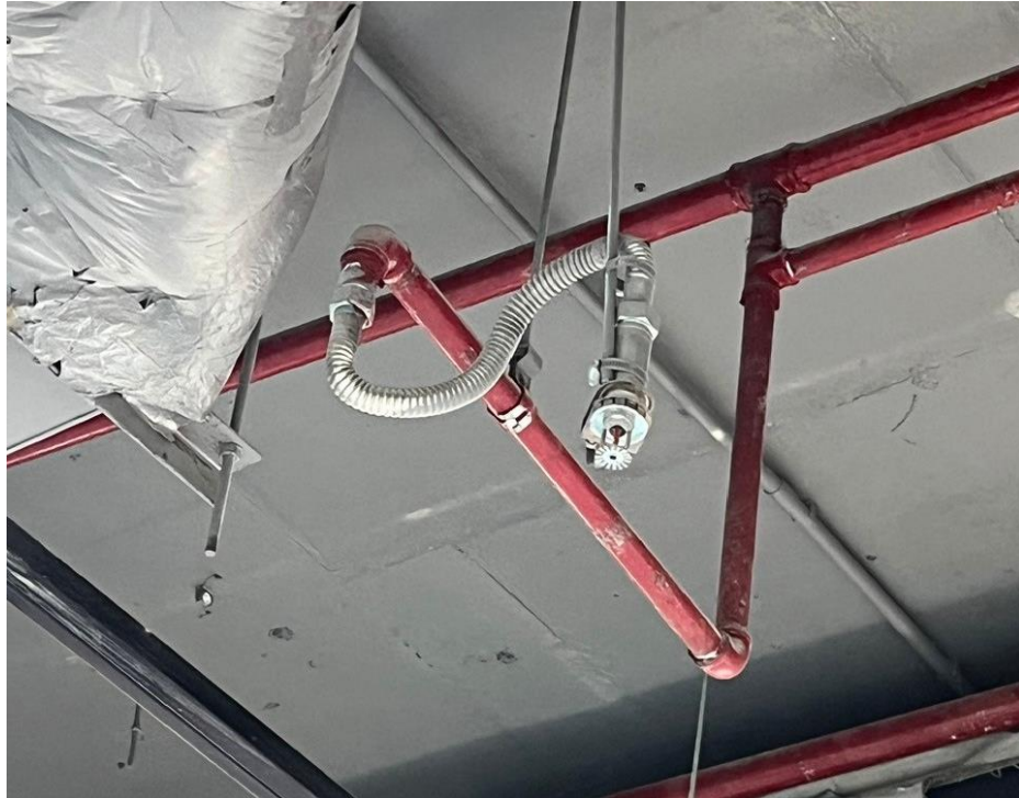
(A flexible sprinkler hose was improperly bent in a mall in Vietnam)
