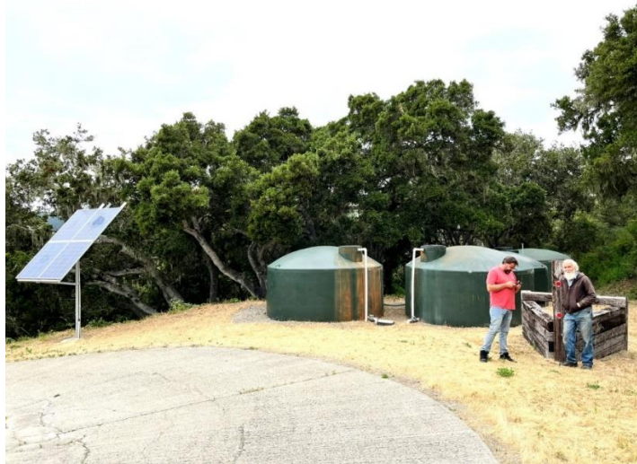
(Water supply system in Camel Valley with storage tanks and a well-pump station. From left to right: Mr. Zachery Vetter, Mr. Larry Weingarten)
