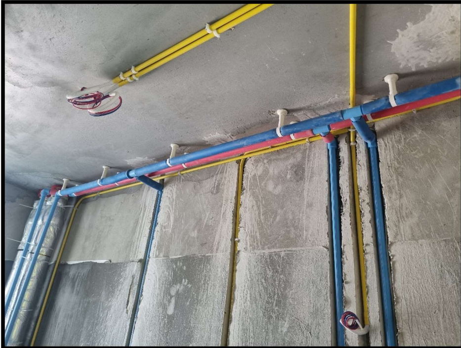
Pre wall installation of MEP services featuring neatly aligned color coded conduits and plumbing using modular clamps
