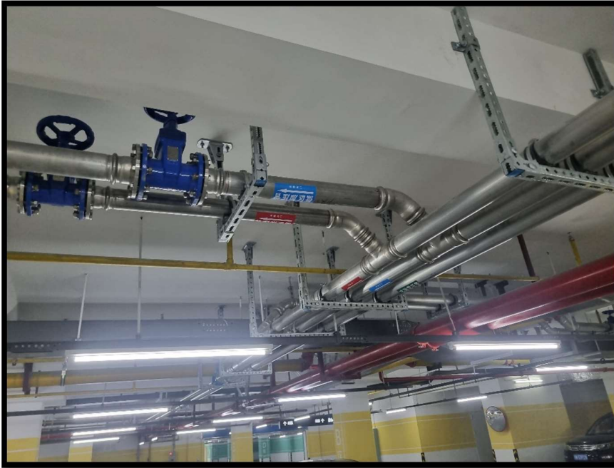
Implementation of SS pipe in high rise residential building 2
