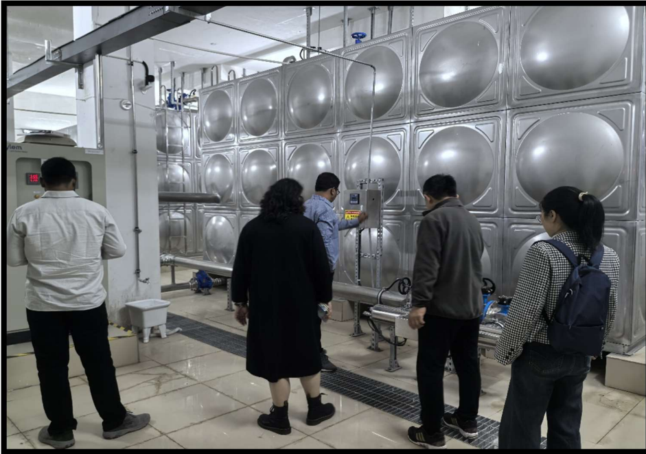
At Imperial Tower, Wuhan Plantroom with SS Buffer Tank and Hydro pneumatic system
