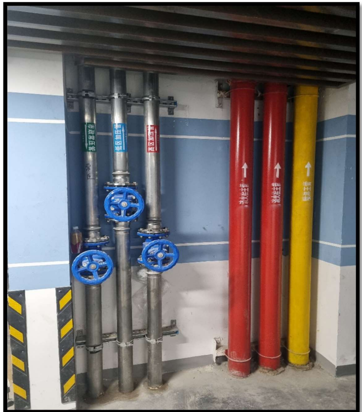
Implementation of SS pipe in high rise residential building
