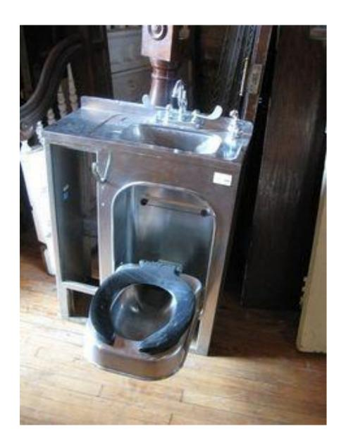
The Patient bed adjacent tip up WC Pan designed for Westmead Hospital by D Creasey & Associates Pty Ltd and approved by Sydney Water. Extract Ventilation bacteria capture from this type of WC pan would be a simple modification. An air ducted quick removable Pan seat and cover as a routine sterilizable item.
