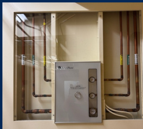
(The local had a extensive area to teach the installation of medical gas to its apprentices, including a life like hospital ward (Above))
