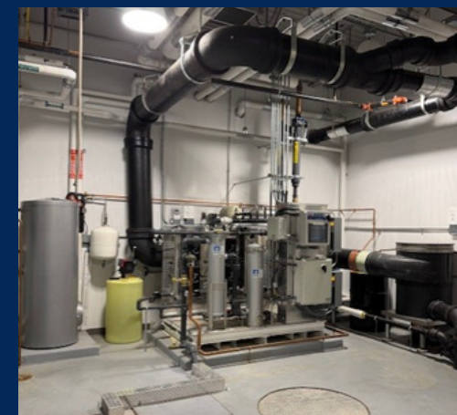
(Above - The training centre is 75% self efficient with its own rain water recycling system and solar PV panels)
