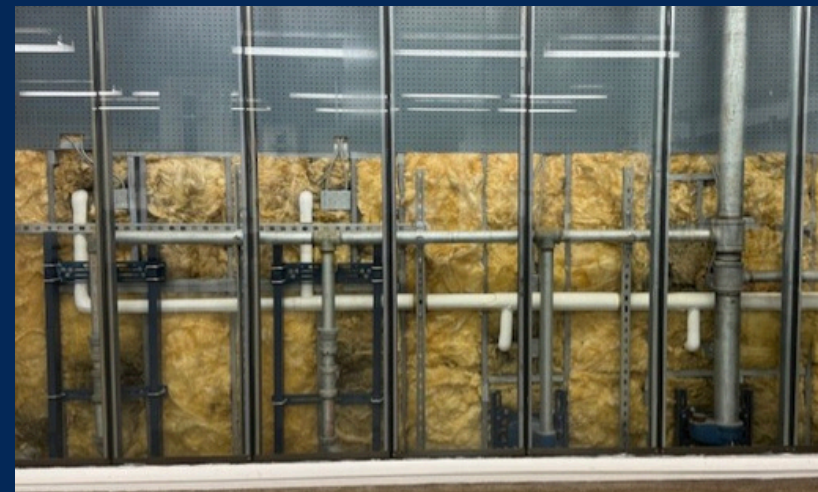
(Above - Waste pipework installation example for a bathroom)
