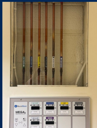
(The local had a extensive area to teach the installation of medical gas to its apprentices, including a life like hospital ward (Above))
