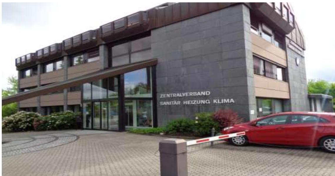
Figure 4 Picture of plumbing, heating and air-conditioning headquarters in St. Augustin
