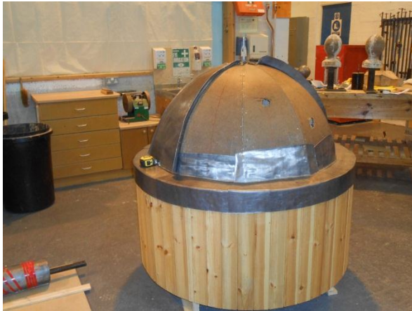
Lead dome being constructed
