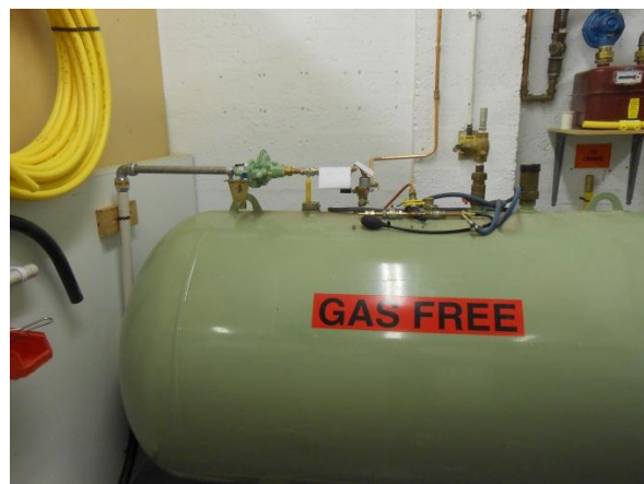
Simulated LPG tank installation
