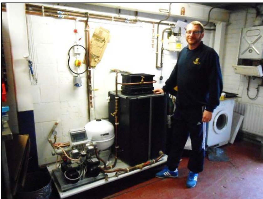
Left - Brett from CK proudly displaying their boosted pressure system
