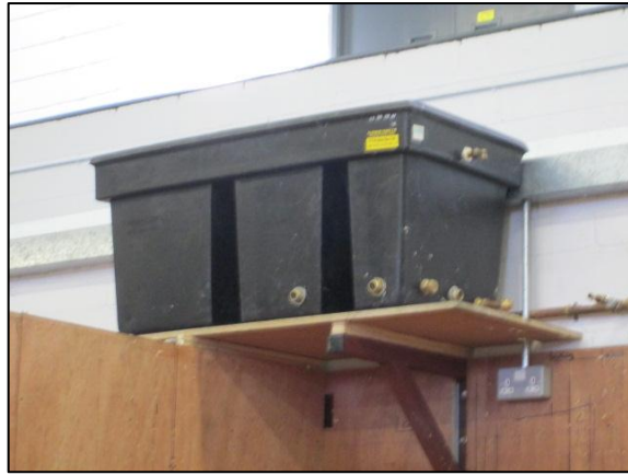
Cold water feed tank for phase 7 project
