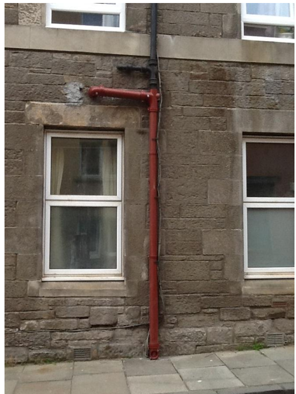
Replacement of cast iron with ductile iron in Edinburgh
