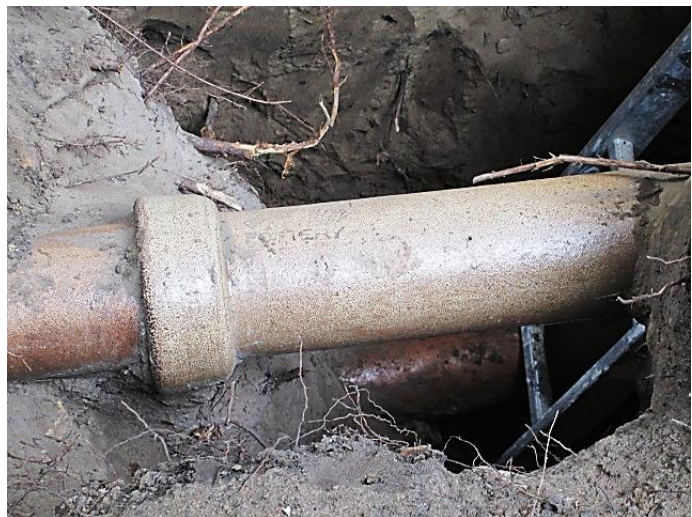
Root intrusion at a property in Bournemouth. The plumber was discussing with the builder whether they should relay or reline.
