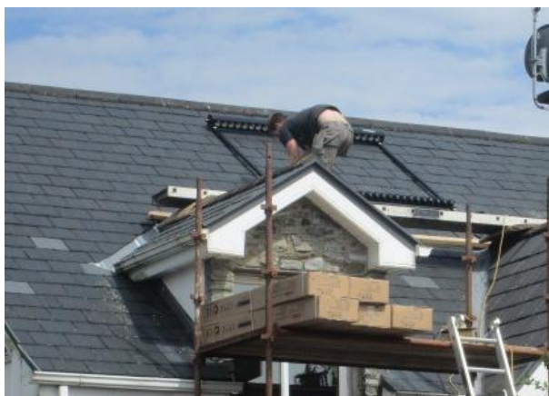
Evacuated solar tubes being installed in Ireland
