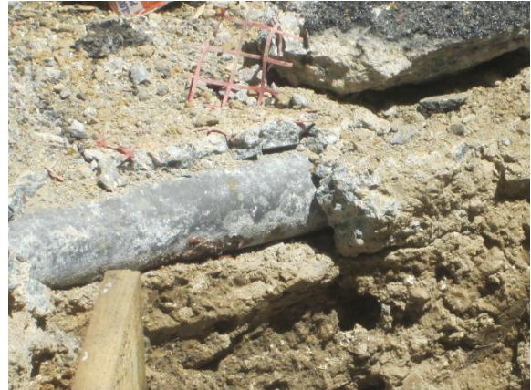
Excavated cast iron main in Paris
