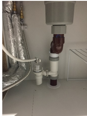
Figure 97 (Blow off trap)
