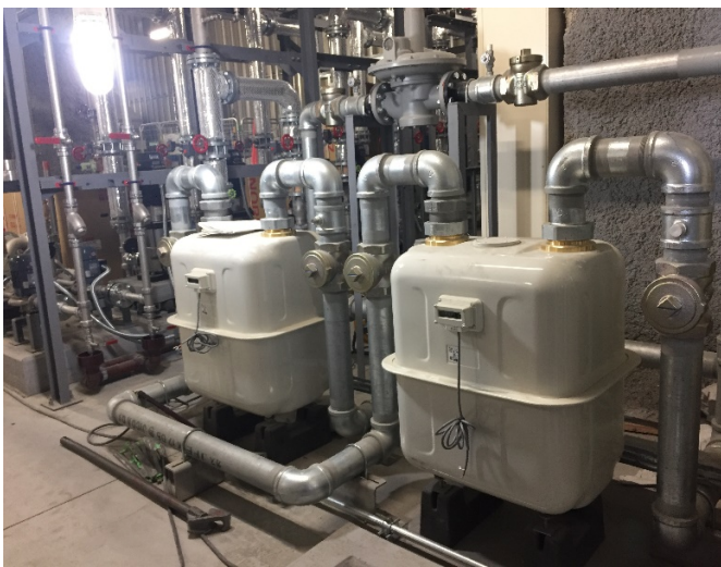
Figure 100 (Gas meters)
