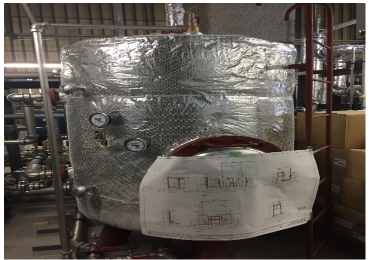
Figure 101 (One of Four calorifiers)
