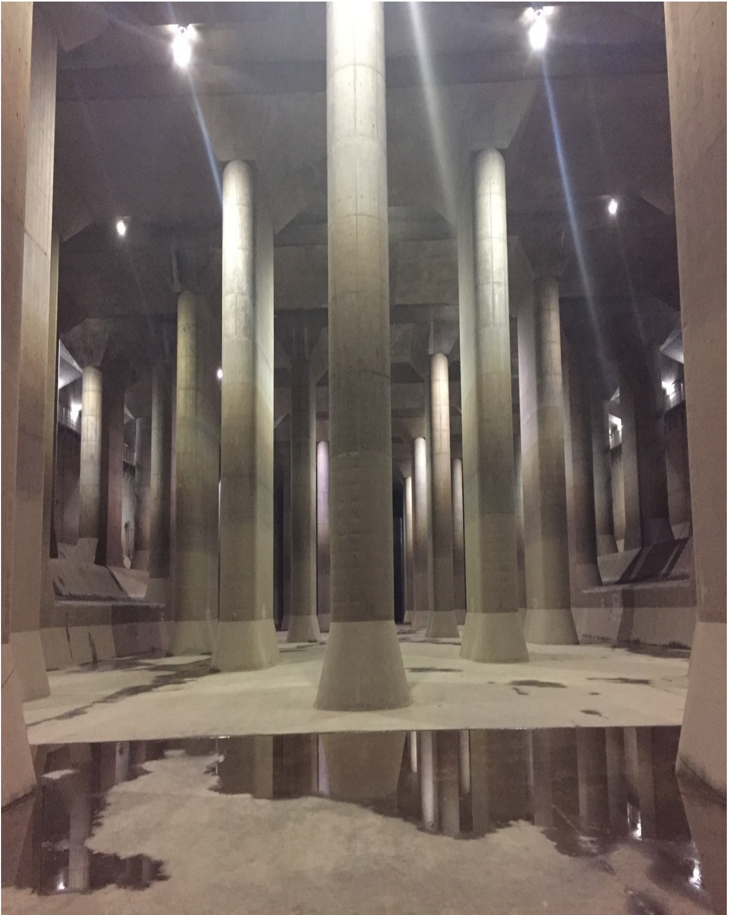
Figure 142 (Inside the pressure adjusting water tank)
