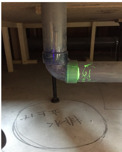
Figure 88 (Fitting with ultraviolet glue)
