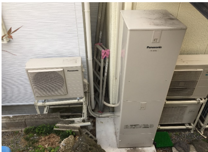
Figure 79 (Panasonic air to water heat pump)
